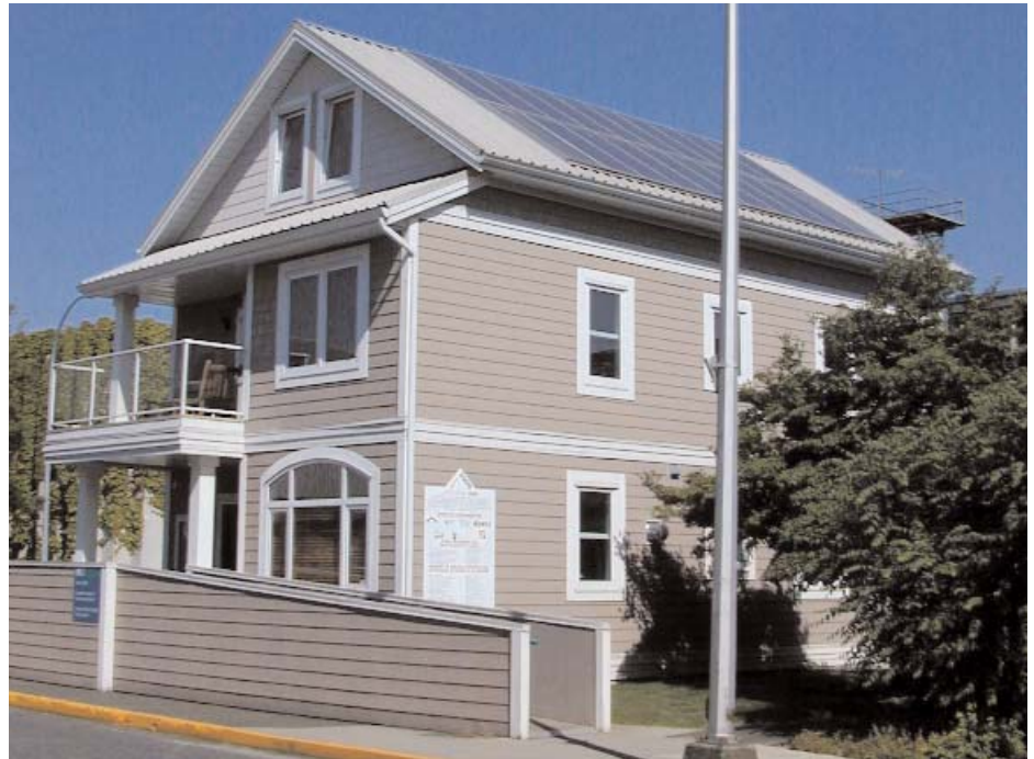
Photo 1: House with a building-integrated photovoltaic roof (BIPV)
